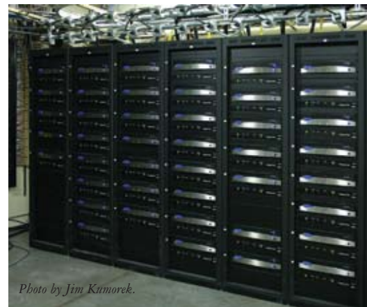
Numerous racks of Crown amplifiers power the PA system at Idlewild.
