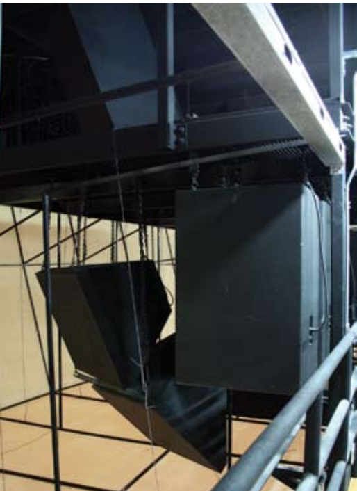
Bill Thrasher of Thrasher Design Group, Inc. designed the PA system around JBL Professional's Precision Directivity PD Series cabinets, with separate boxes handling the mid- and high-frequencies, another group of cabinets for the bass, and a set of subwoofers for additional low-end.
